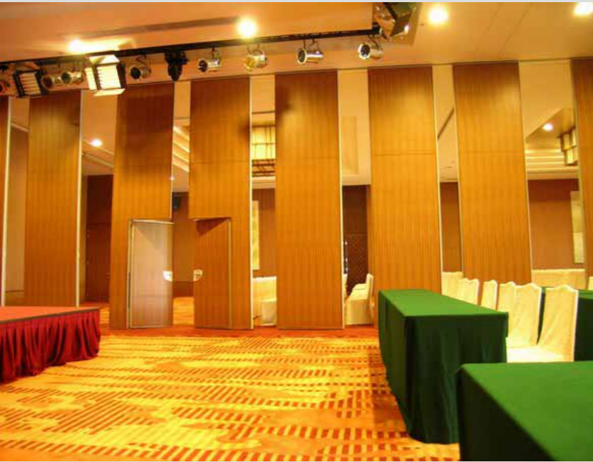
The press bar automatically conceals when the door is opened
