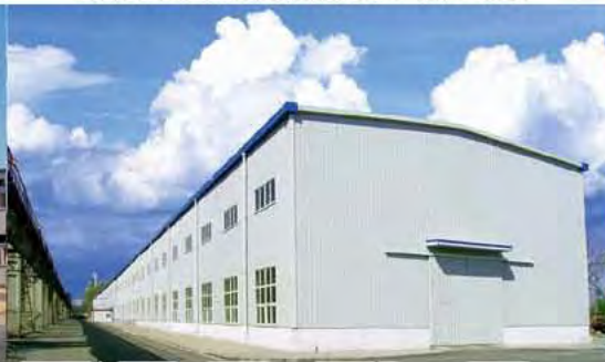
LIGHT STEEL STRUCTURE BUILDING
