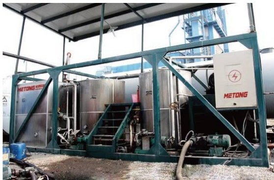
Guizhou construction site
