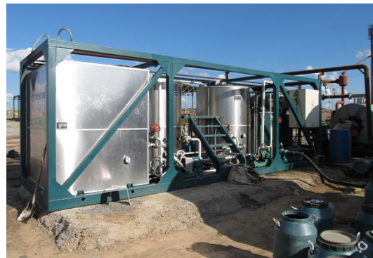
Inner construction site
