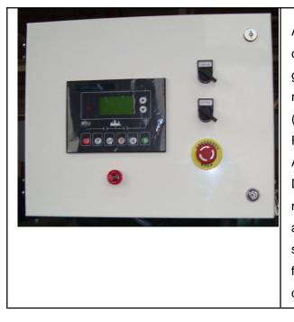
Automatic Control Panel is the basic configuration for nobody on duty controlling generator. This kind of panel can accept the remote Start/Stop signals. (Controlled by ATS) Features: adopted Chinese producing, Auto control system, with large LCD, Display in English (or CHINESE) to show the menu. With Auto Control Panel .generator are of various functions such as auto/manual stop (Emergency Stop), programmable plugs for input and output detected data, symbols diagram will show in the LCD, etc.
