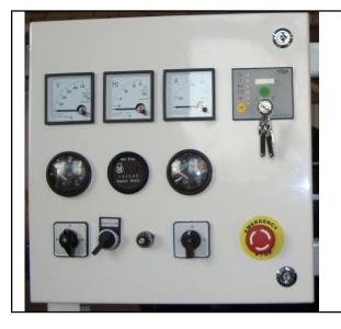
Standard Control Panel is the basic configuration for normal operation and usage. It is of some advantage such as easy to operate various function and well protection. Operative buttons such as Turn On, Per-heart. Starting, Stop (Emergency Stop) on the panel .while malfunction occurs, control panel will stop the generator and also alarm with light or buzz.
