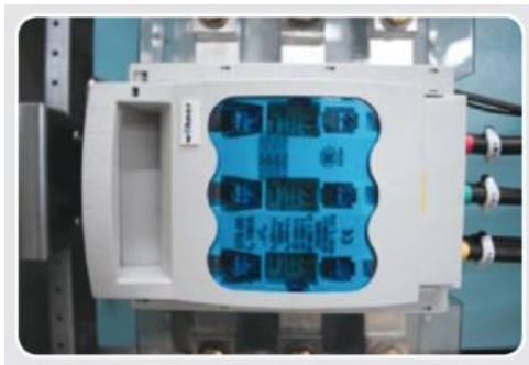
Disconnecting switch
